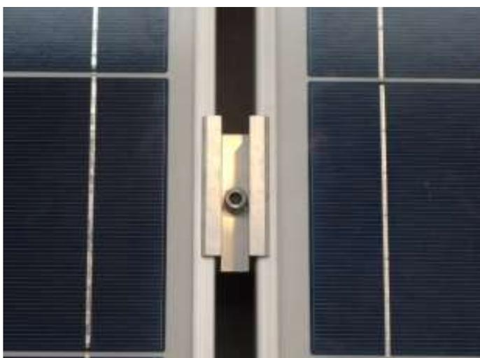
**Clamp type: ZETA** For this clamp type, it is necessary to use screws which characteristics are :  $\varnothing$  8mm, length 25mm
